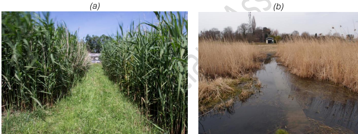
Figure 3.4 Examples of maintenance impacts on access paths to wetland cells, (a) well maintained grass access path (Photo credit D Naismith), (b) inundated wetland with water connecting two independent cells and unsafe pathways. Photo credits: (a) Dave Naismith and (b) G Dotro.
