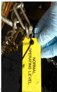
Figure 3.3 Example of operational water level checks, (a) Best practice has tags to clearly indicate where the normal operating water level setting should be for a HF or SF cell, (b) Rodding of effluent collection pipe in a HF cell. All pictures credit NbS Future/G Dotro.
